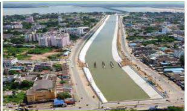
Taladanda Main Canal
