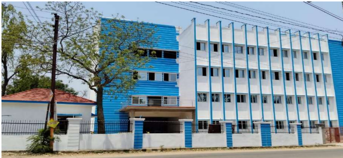
Construction of Commercial office
