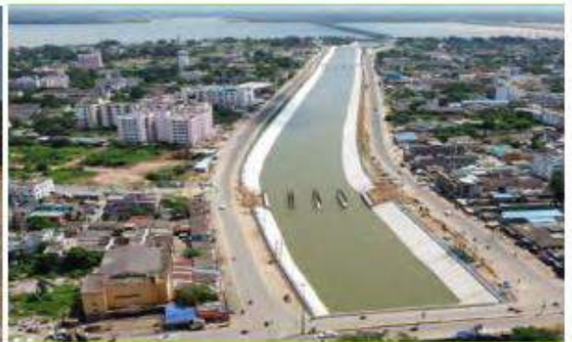
Taladanda Main Canal
